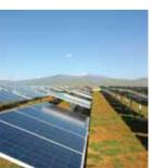
Project Site: Macedonia Load Capacity: 8MW Material: hot dip galvanized steel Q235B Client: Intebako doo Time of installation: March, 2011 Solution: G-A Ground mounting
