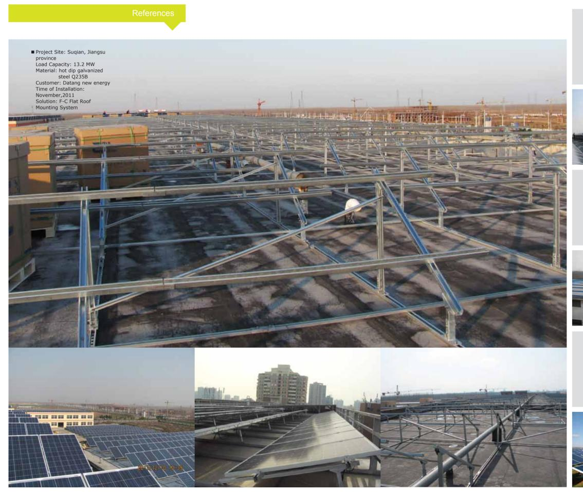
Project Site: Suqian, Jiangsu province Load Capacity: 13.2 MW Material: hot dip galvanized steel Q235B Customer: Datang new energy Time of Installation: November,2011 Solution: F-C Flat Roof Mounting System -
